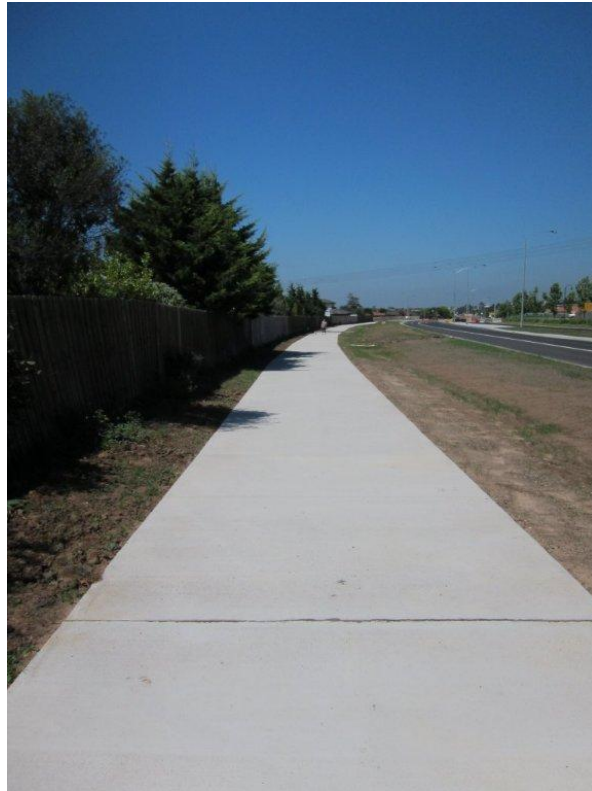
Figure 3. E-Crete Footpath (Calder Freeway Interchange)
